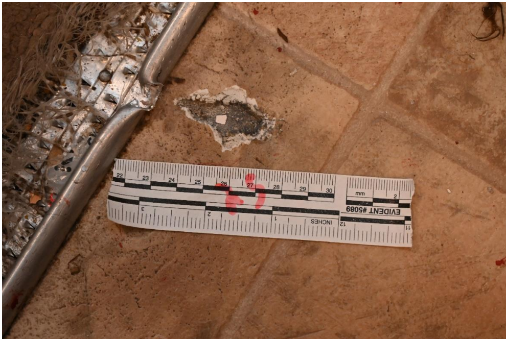
Figure 6: Ballistics damage to Mr. Maclean's floor consistent with being fired by Mr. Maclean.
